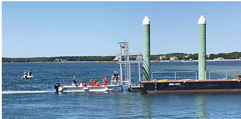
“The opportunity to work in the clean-energy industry is great for our members,” said Dave Borrus, Pile Drivers and Divers Local 56 business manager. (Courtesy: Massachusetts Maritime Academy)
