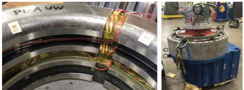
Figure 2: Planet-bearing instrumentation (left) and partially assembled gearbox (right). Photos by Jonathan Keller, NREL 36522 and 36512.
