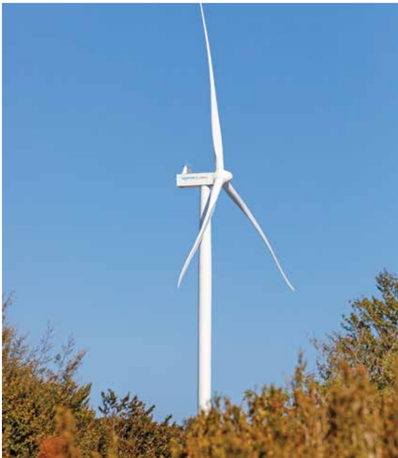
The 71-meter blade on the SG 4.X platform integrates aerodynamics and noise reduction features (Courtesy: Siemens Gamesa)
