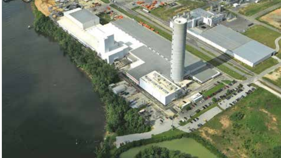
The tower that is part of the manufacturing process is the tallest building in South Carolina at 427 feet. (Courtesy: Nexans)
