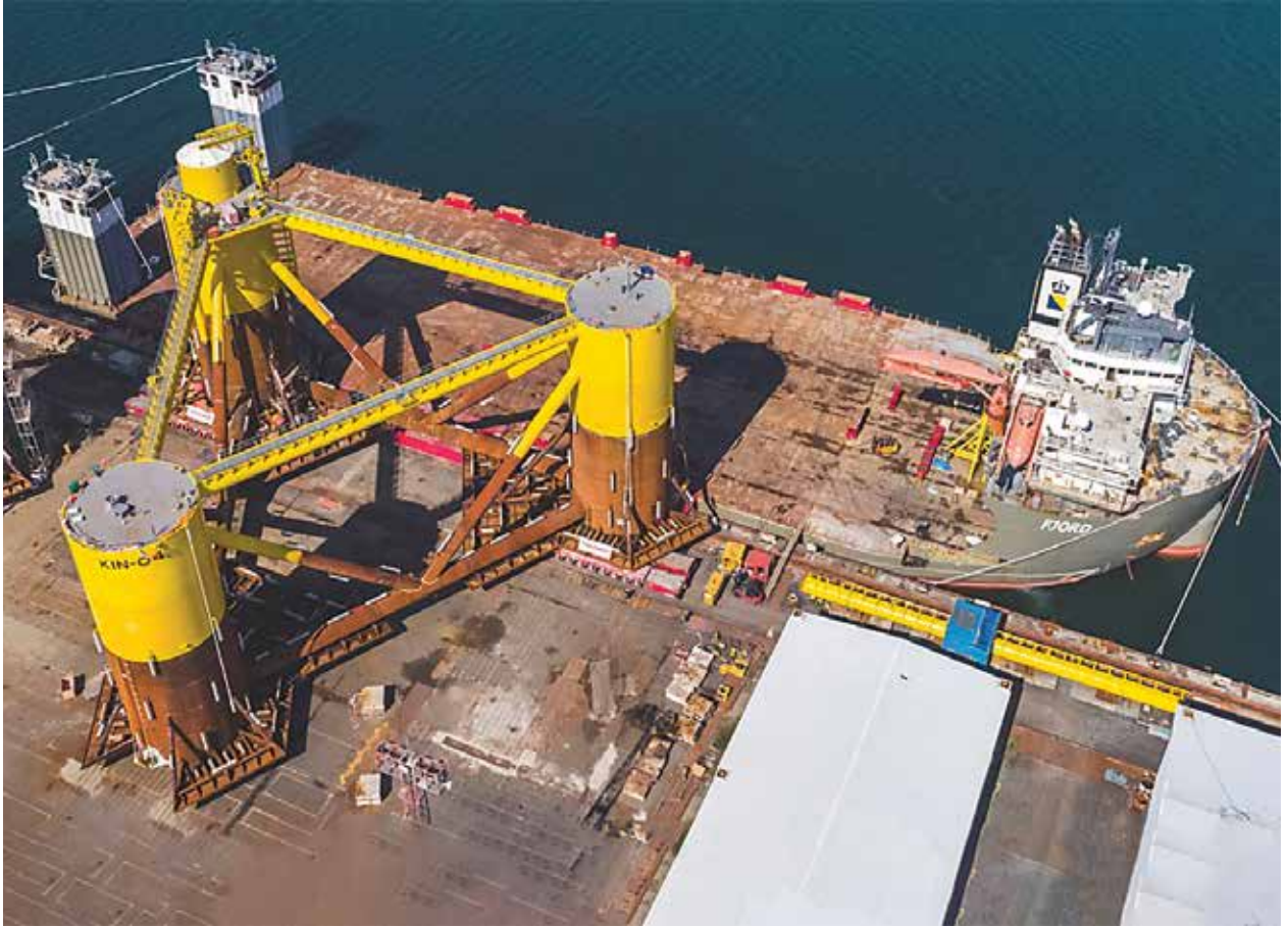
Load-out at Kincardine Offshore Wind Farm. (Courtesy Mammoet)
