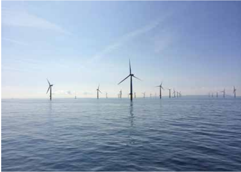
Gwynt-y-Môr is a 576-MW offshore wind farm off the coast of Wales. (Courtesy: Fisher Renewables)
