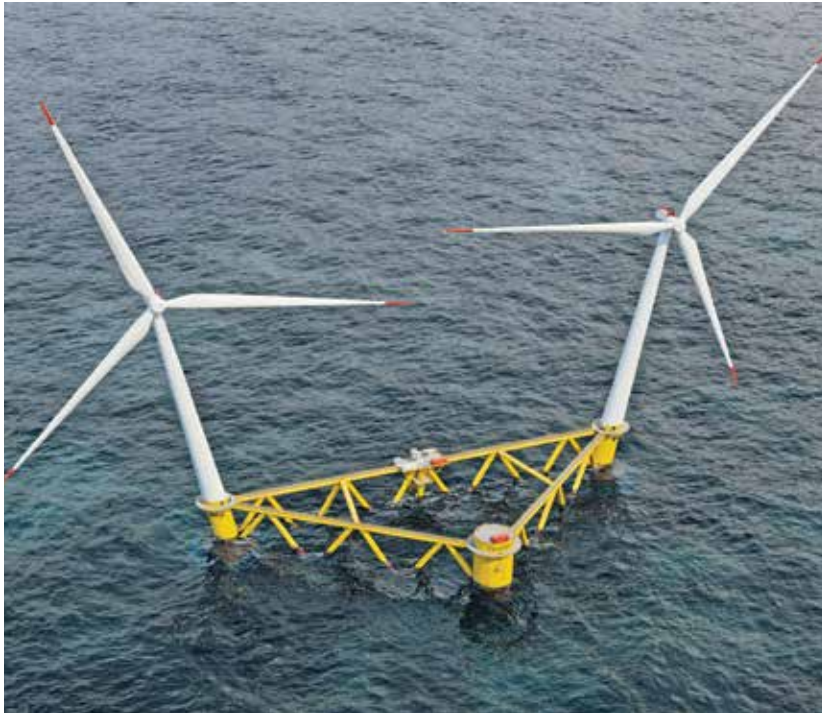
DNV considers the TwinWay concept feasible for further development toward a full-scale demonstrator. (Courtesy: DNV)
