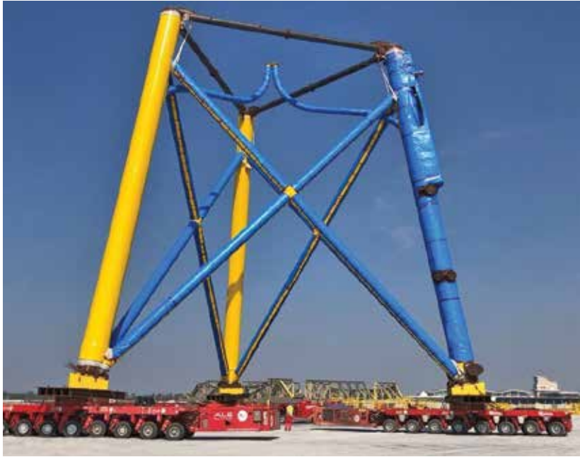
Upper and lower jackets were sat on top of the custom support saddles that were used on the self-propelled modular transporters to transport both pieces between assembly stations. (Courtesy: Mammoet)
