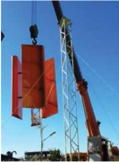
Figure 13: Crane lifting the top of the wind turbine.
