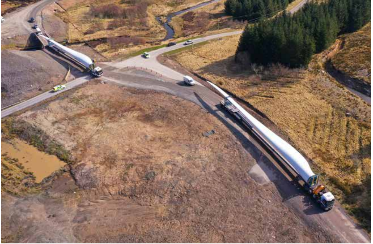
Phase 1 of the Kennoxhead Wind Farm is now completed. (Courtesy: Collett)
