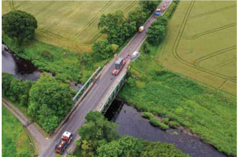
Moving an 80-metric-ton transformer across Glassford Bridge presented a challenge. (Courtesy: Collett & Sons)
