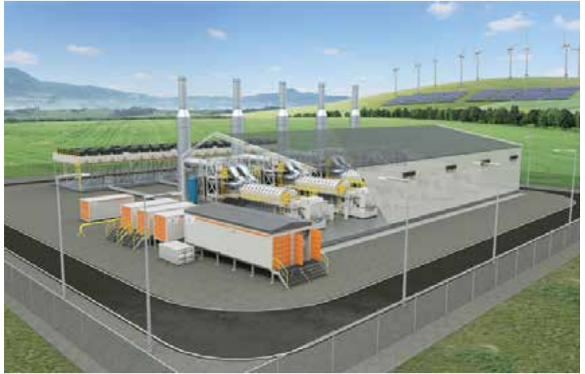
The Wärtsilä 315G contains a cost-efficient plant construction design, based on prefabricated power plant modules. (Courtesy: Wärtsilä)
