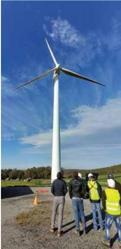
Perceptual Robotics engineers flew an M300 drone to autonomously inspect a G47 wind turbine. (Courtesy: Perceptual Robotics)
