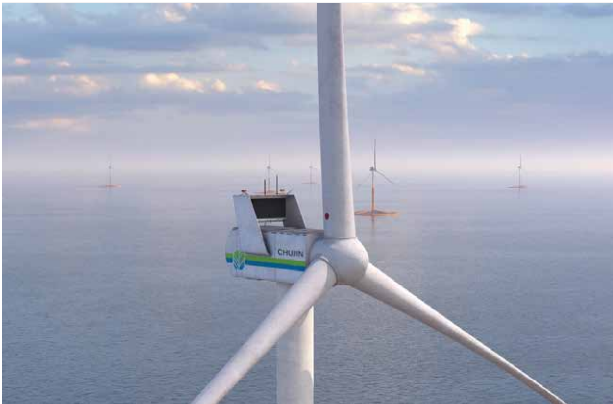
When the Chujin plant is finished, it will be South Korea's largest commercial-scale offshore wind farm. (Courtesy: DNV)
