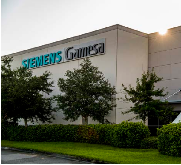
The Wind Academy facility located in Orlando, Florida. (Courtesy: Wind Academy by Siemens Gamesa)
