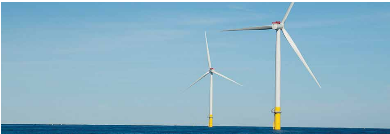
These two wind turbines, currently in operation, were the first installed as part of the Coastal Virginia Offshore Wind commercial project. (Courtesy: Dominion Energy)
