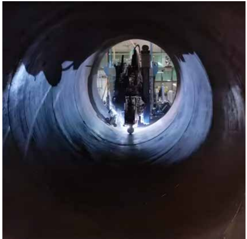
Keystone's tapered spiral welding process brings the speed, quality, and consistency of automated manufacturing to wind-tower manufacturing. (Courtesy: Keystone Tower Systems)
