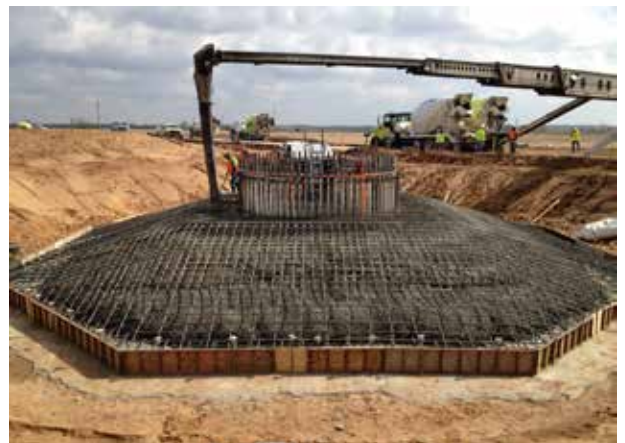
Photo 1: -When constructing a typical wind turbine foundation, concrete is poured over steel reinforcement before being cured and backfilled. (Courtesy: Barr Engineering Co.)
