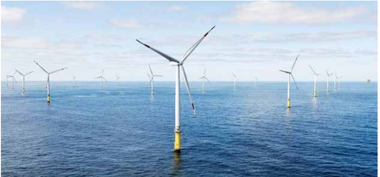
New Jersey has reached an agreement for Ocean Wind to deliver 1.1 GW of offshore wind generation. (Courtesy: Business Network for Offshore Wind)
