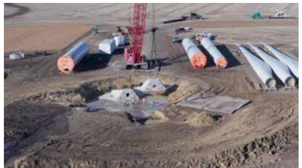
Photo 2: Pre-cast concrete sections are lifted into position at the Palmers Creek Wind Farm in Granite Falls, Minnesota. The sections will be post-tensioned and then backfilled before tower erection begins. (Courtesy: Barr Engineering Co.)
