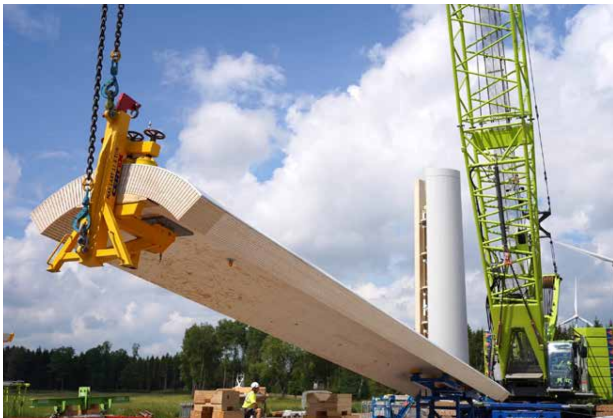
The wood technology company Modvion is building a 105-meter wind-turbine tower made of wood, the tallest of its kind, in Sweden. (Courtesy: Modvion)
