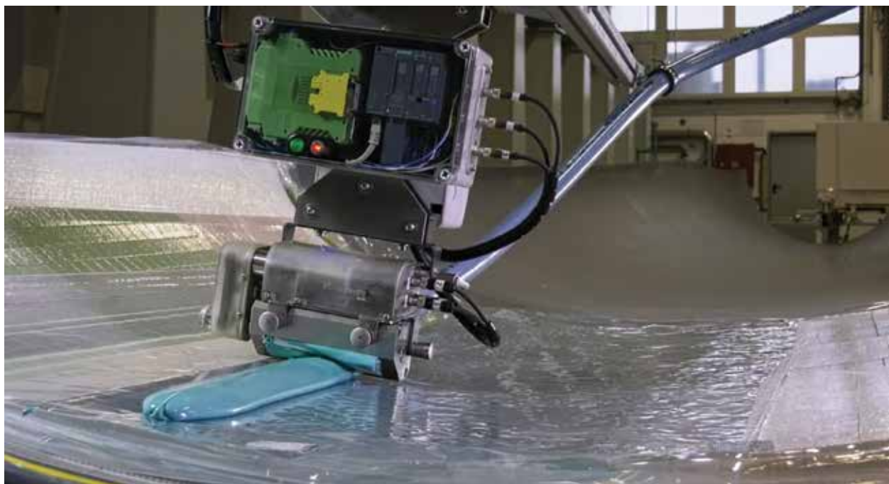
Automated application of bonding agent in the blade. (Courtesy: Siemens)
