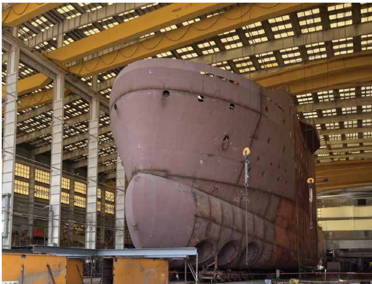
A closeup of the ECO Edison — the first American-built Service Operation Vessel for offshore wind — under construction in Houma, Louisiana, earlier this summer. (Courtesy: Business Network for Offshore Wind)
