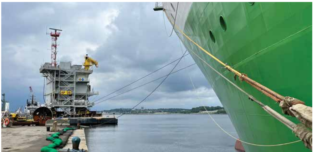
The first American-made offshore wind substation at ProvPort in Providence, Rhode Island readying for installation. (Courtesy: South Fork Wind)
