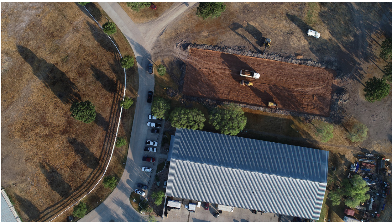
TDI-Brooks breaks ground and begins construction of a new expansion building at TDI's headquarters in College Station, Texas, 90 minutes north of Houston. (Courtesy: TDI-Brooks)
