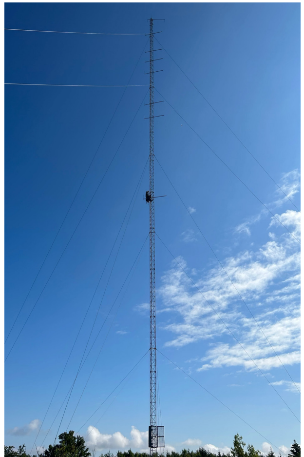
A MET tower installation at wind-farm development. (Courtesy: EverWind Fuels)
