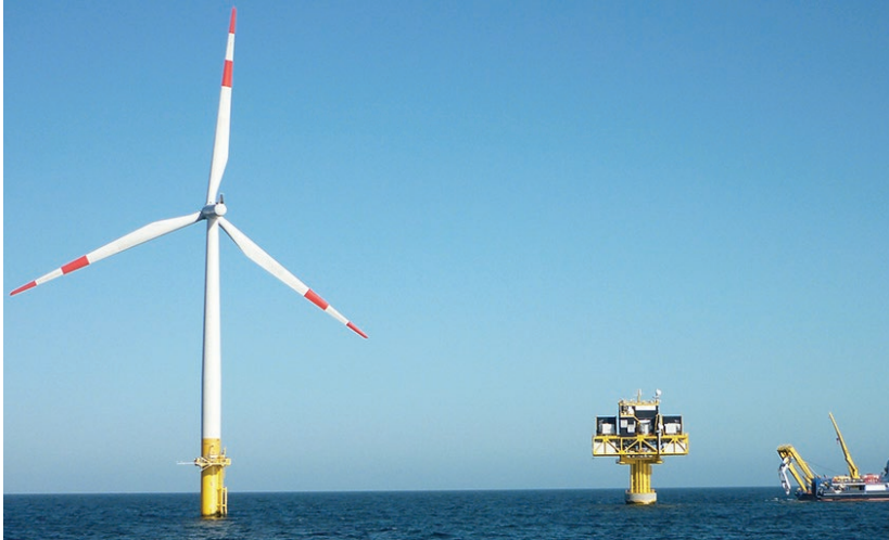
A collaborative industry effort has brought together 38 participating companies to tackle challenges associated with floating offshore substations. (Courtesy: DNV)
