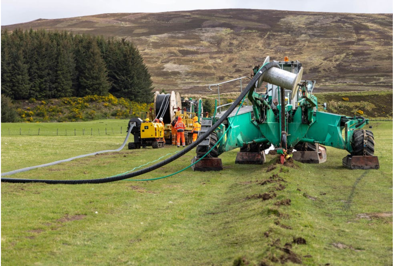
The Eco Cable Protect wrapping system applies an extruded high density polyethylene mesh wrap to power cables, which delivers reduced project costs. (Courtesy: McGowan Environmental Engineering)
