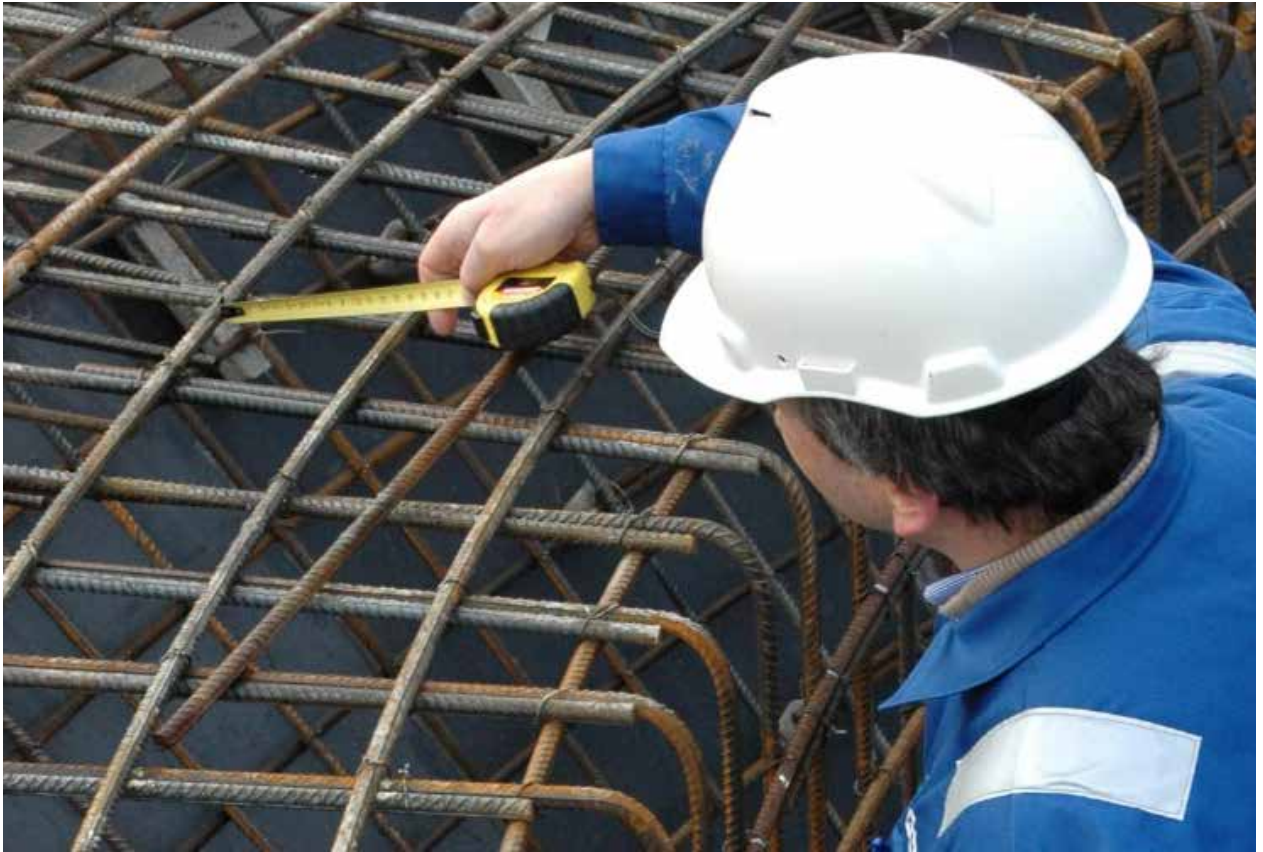
The joint industry project encompasses concrete structures, geotechnics, and floating technologies and welcomes additional partners. (Courtesy: DNV)
