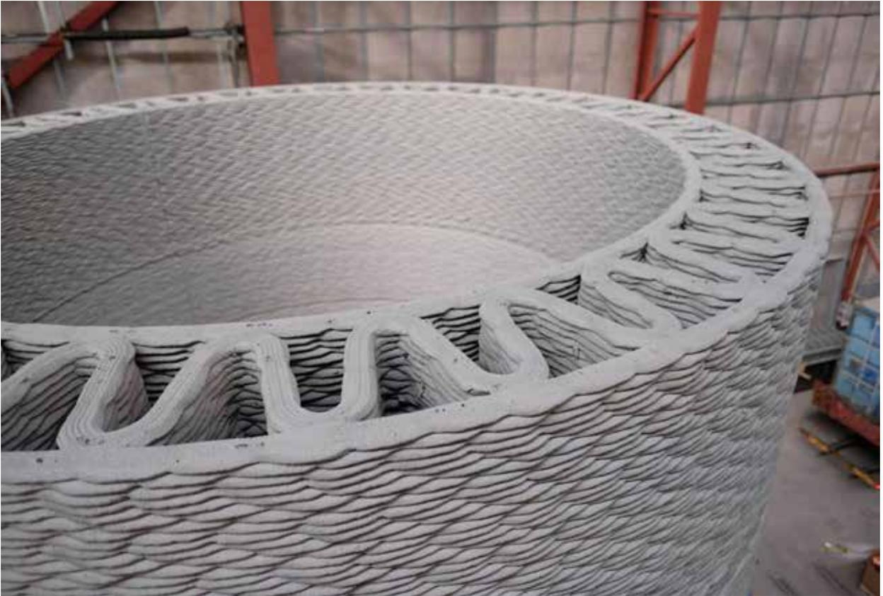
A prototype of a wind-turbine base 3D printed from concrete. (Courtesy: GE)
