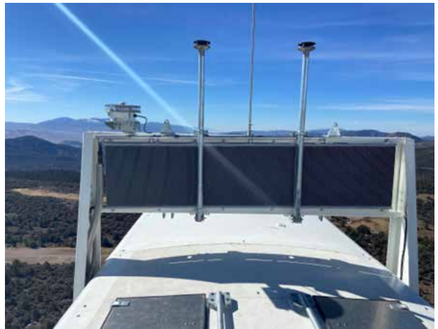
Condenser coil on the nacelle of a wind turbine for a loop thermosyphon. (Courtesy: ACT)
