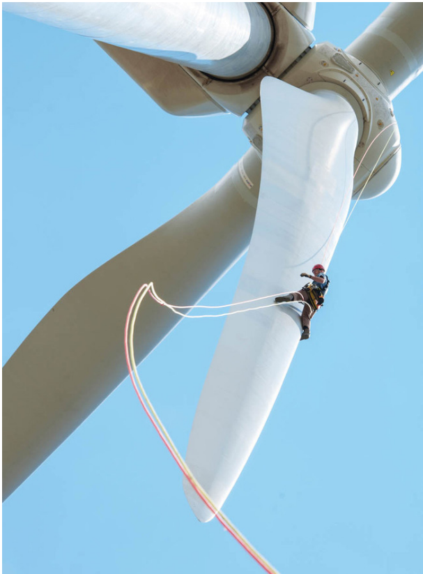
Traditionally, LPS inspections have required teams of certified climbers scaling turbines, a time-consuming and hazardous task. (Courtesy: Dennis Schroeder/NREL)
