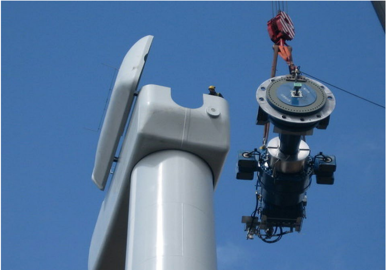
This shows the wind turbine gearbox installation of the rotor shaft and disk brake assembly. (Courtesy: Euro ns TestOil)
