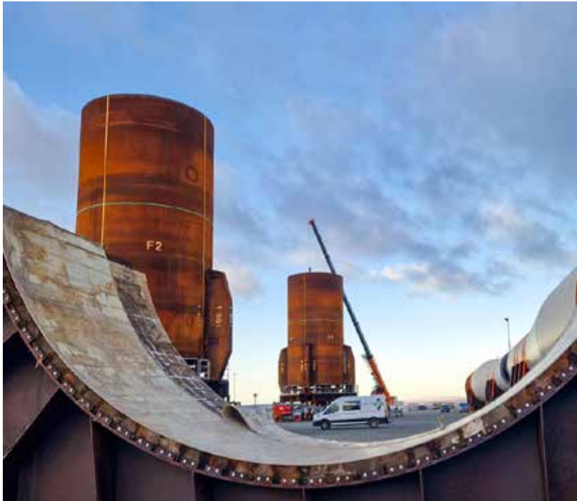
Inch Cape Offshore has awarded Aventus with a contract for the delivery of foundation completion activities on its 1.1-GW offshore wind farm. (Courtesy: Aventus Energy)
