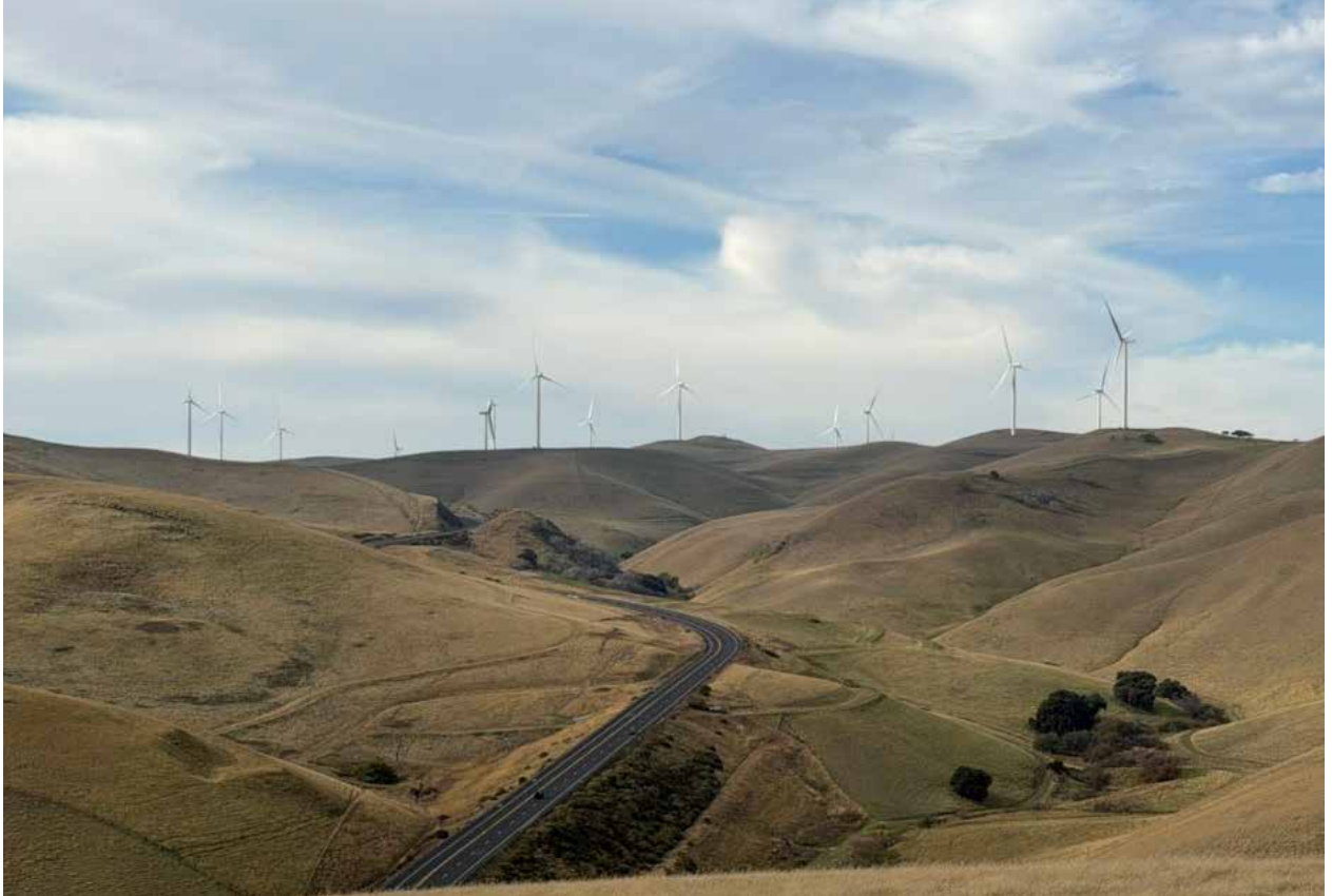
Buena Vista Wind Farm in California has been refurbished with blade enhancements, modernized control equipment, and more. (Courtesy: DWT)
