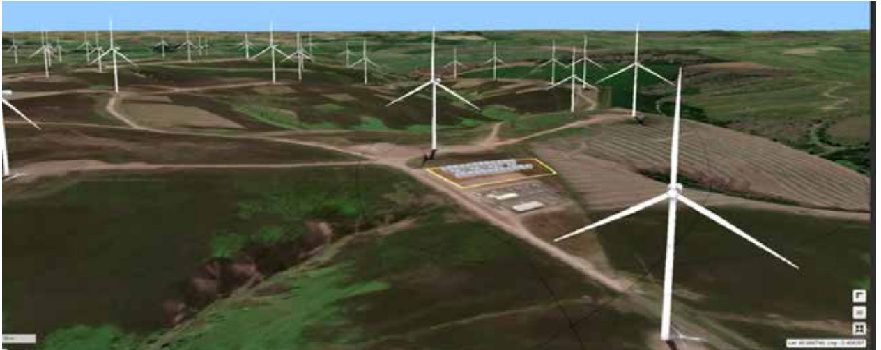
Youwind has launched BESS, a Battery Energy Storage System module. (Courtesy: Youwind)
