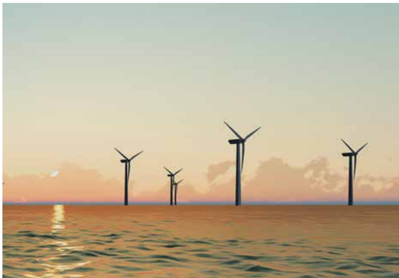
North East England’s offshore wind cluster is moving forward with the next phase of offshore leasing. (Courtesy: Energi Coast)
