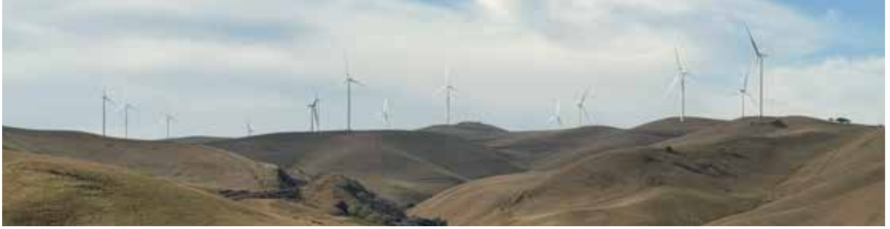
Buena Vista Wind Farm has been refurbished with blade enhancements and modernized control equipment. (Courtesy: DWT)
