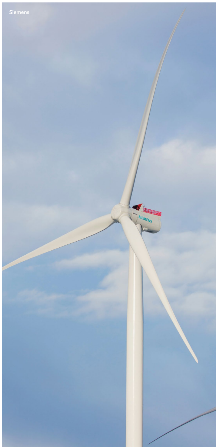
Two prototypes were installed in Osterild, Denmark, to run comprehensive product tests of the 7-MW offshore wind turbine.
