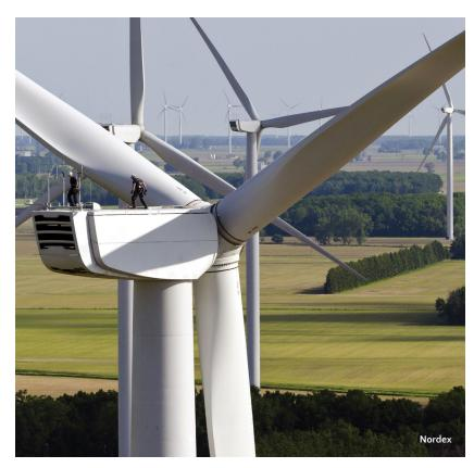
N117/2400 Gamma (2.4 MW) wind turbine
