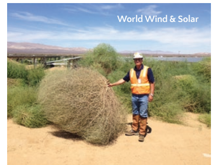
An example of a tumbleweed on a construction site.
