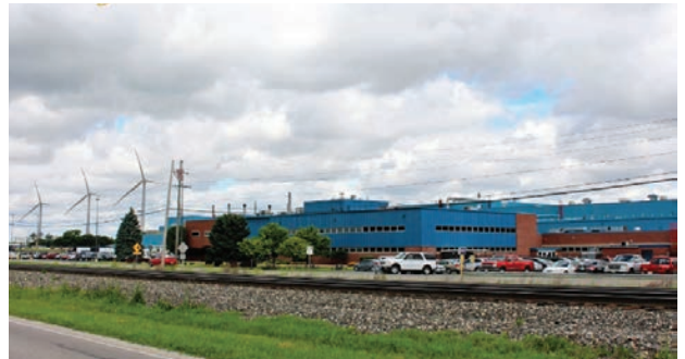
Rendering of what the Marion Wind turbines would look like once completed. (Courtesy: Whirlpool Corporation)
