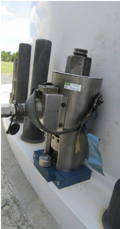
Load-indicating washer being installed during base-bolt tension check. (Courtesy: Torkworx)
