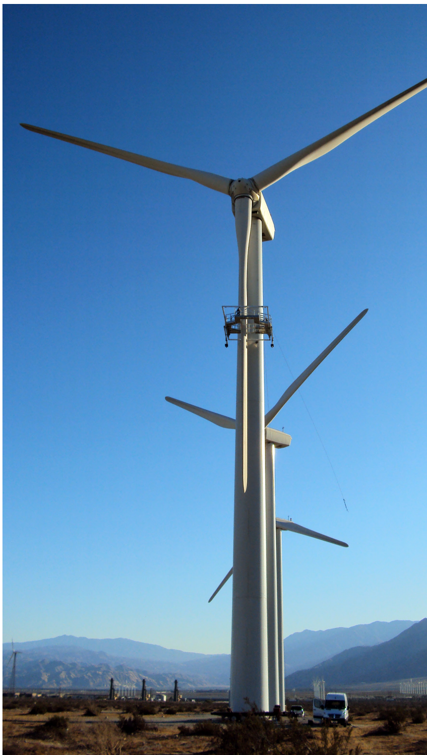
BS Rotor Technic USA has several years of experience and uses its technical knowledge and expertise in the service and repair of wind-turbine rotor blades. (Courtesy: BS Rotor Technic USA)
