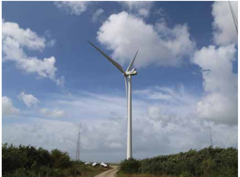
The Copenhagen Wind Project will use 40 Vestas V110 2.0MW turbines such as the one pictured here. (Courtesy: Vestas)
