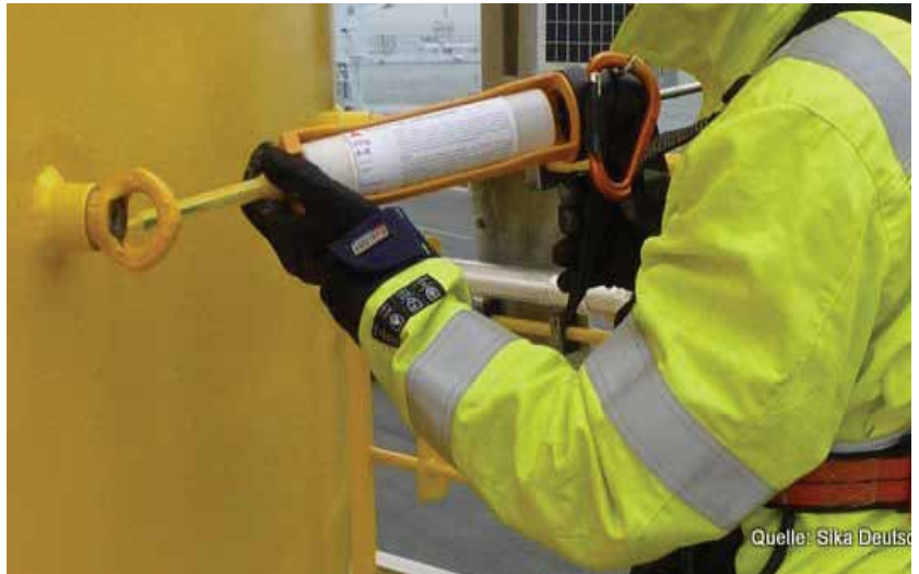
SikaCor SW-1000 RepaCor is applied. (Courtesy: Windsourcing.com)
