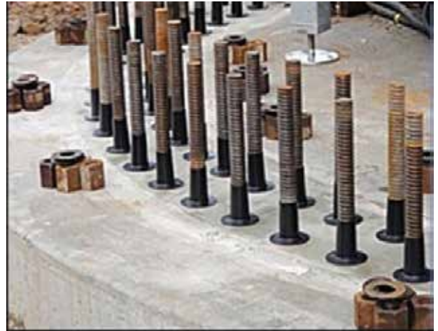
Grout sleeves are useful for over-wintering foundations. (Courtesy: NTC Wind Energy)
