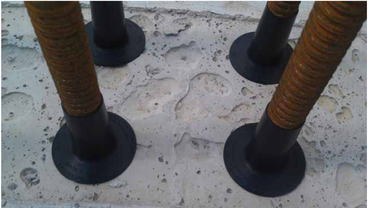
Foam rings are still predominantly used today and the process is no more sophisticated than it was at the beginning. (Courtesy: NTC Wind Energy)
