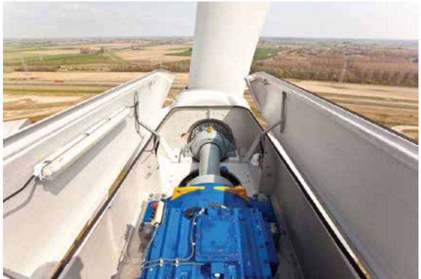
A wind-turbine gearbox operates in uniquely severe conditions. These include heights of up to 350 feet above the ground, heavy and varying loads from strong winds, and exposure to contaminants such as saltwater in an offshore environment.
