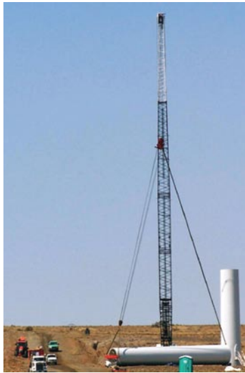
Fig. 5: Erecting tower base with wheel-mounted crane.
