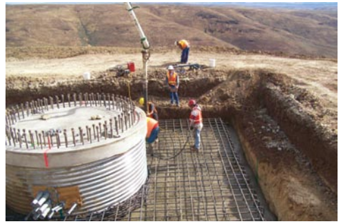
Fig. 3: Pumping concrete collar around completed foundation in soft soil.
