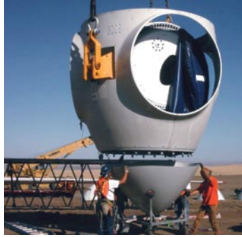
Fig. 4: Assembly of nacelle in marshalling yard.
