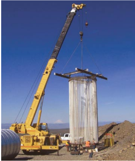
Fig. 2: Lowering assembled bolt cage.
