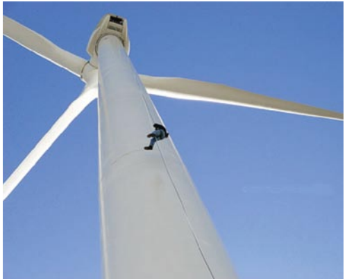
Fig. 2: Ascending the tower for O&M can be challenging and exhausting (NREL).
