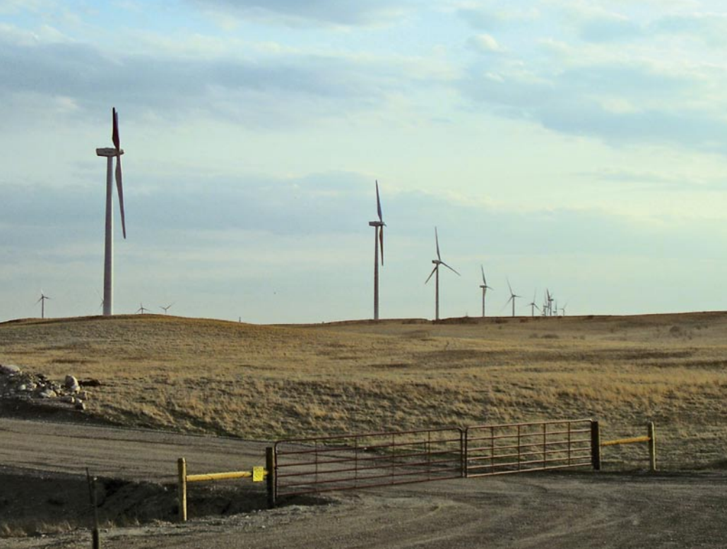
Fig. 2: Site access gate for the Tatanka Wind Farm in North Dakota.
