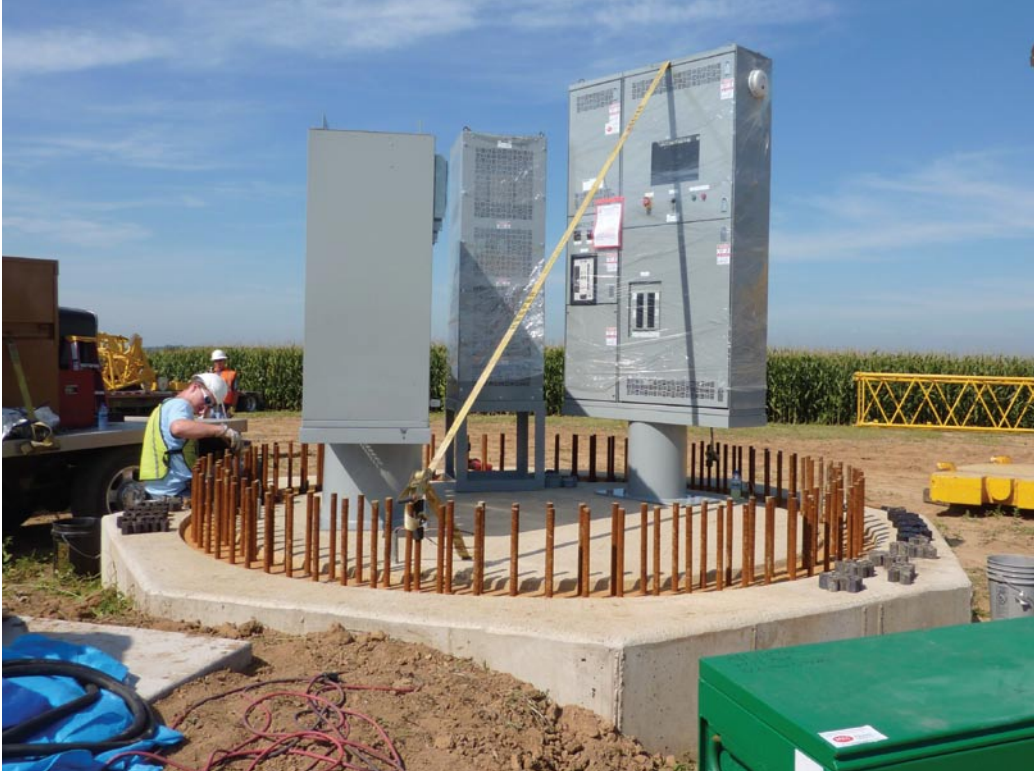
Fig. 3: Construction project installing a 900KW wind turbine converter.
