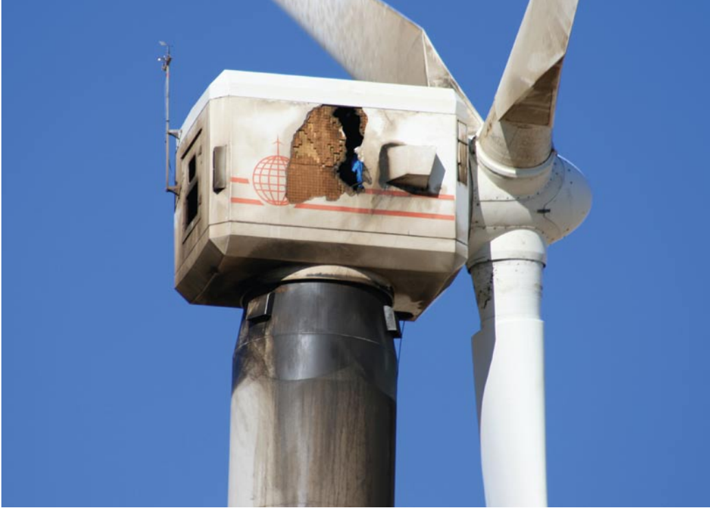
Fig. 2: This fire was caused by a blown coupling.
