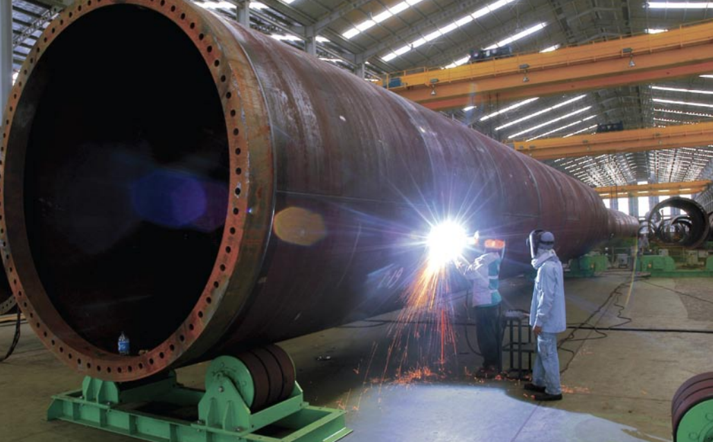
Fig. 2: A worker prepares a tower section.
