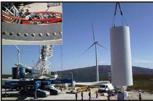
Fig. 3: i-Bolt technology drastically reduces time, effort, and money compared to conventional inspection techniques.
