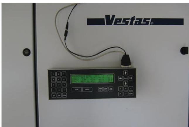
**Fig. 4:** With a control box maintenance is quicker and easier because the wind turbines can be controlled directly from the powerhouse by a portable control panel (Vestas).
