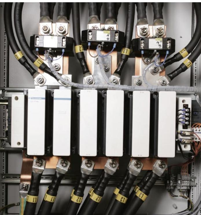
**Fig. 2:** The grid coupling contactor, handling the switching processes of the main switch, can generally prevent damage and increase turbine availability (GE).
