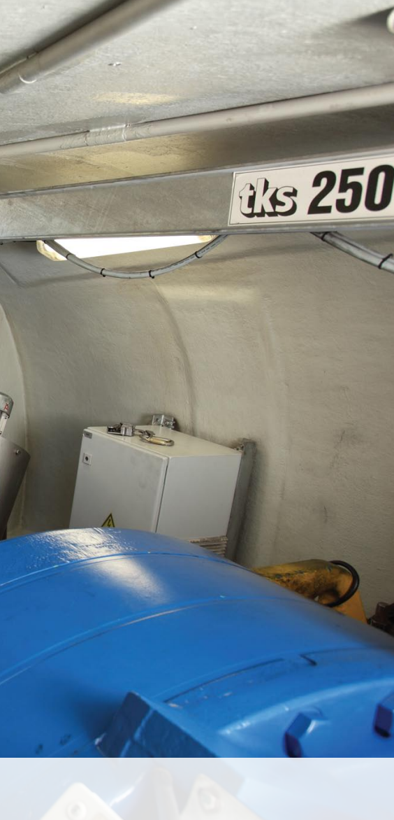
Fig. 1: It's common for technicians to carry a bag with more than 100 tools going from turbine to turbine. The last thing you want is to find one missing.
