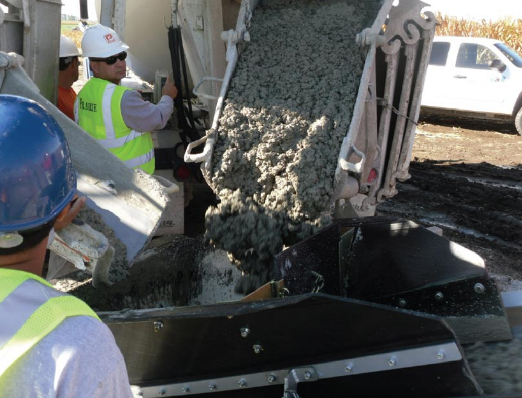
Fig. 5: Concrete is loaded from the truck into the material delivery system.
