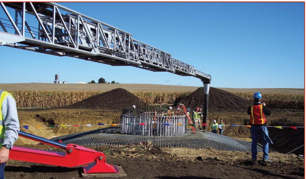
Fig. 3: The telescopic conveyor belt carries material to the foundation site.
