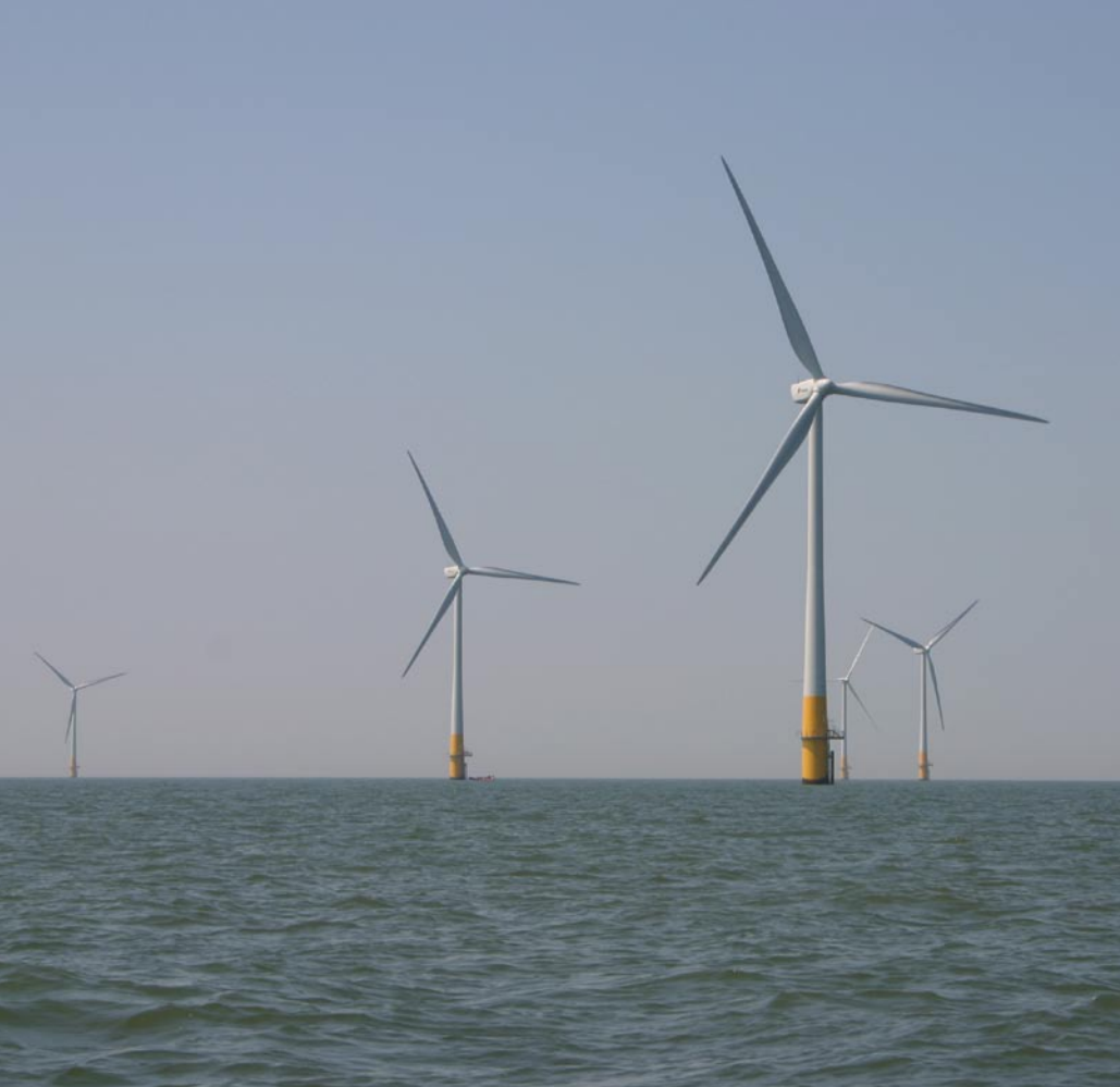
Fig. 2: Rambøll's structures penetrate the seabed up to 30 meters and must withstand the constant pounding of tides, waves, and currents, in addition to the loads of the wind tower itself.
