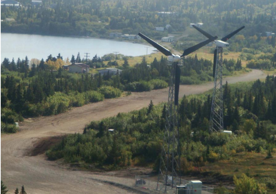
Fig. 2: The two Vestas V-17 turbines rated at 90kW each on 85' lattice towers with 56' rotors, and 180 kW of connected wind capacity were remanufactured by Halus Power Systems.
