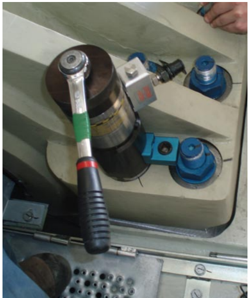
Fig. 2: A Torcup tensioning device in use.
